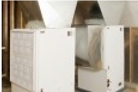
Figure C1. Air recirculating unit
