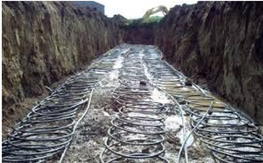
Figure 5. Single “slinky “ pipe system
